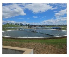
Following the aeration tanks, the wastewater passes through a final clarifier section to capture the biological organisms that settle in the final clarifiers. These biological organisms that settle are returned to the activated sludge aeration tanks.
